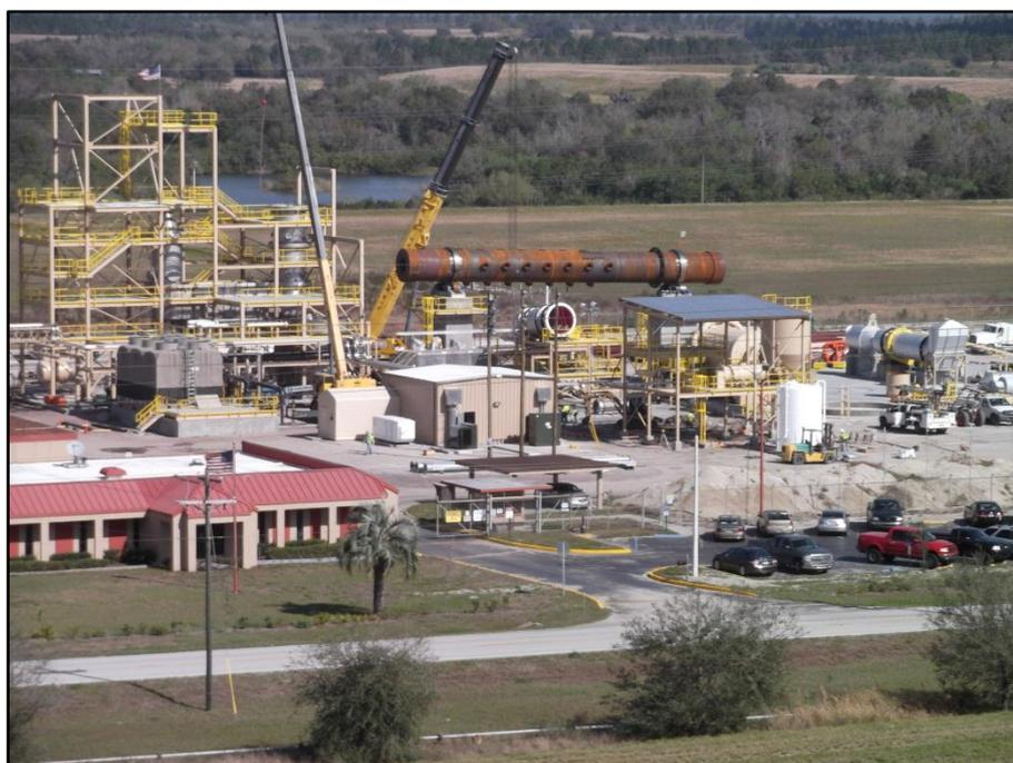
*Figure 4: JDCP Demonstration Plant under construction, ported kiln now in place, January 2013*
